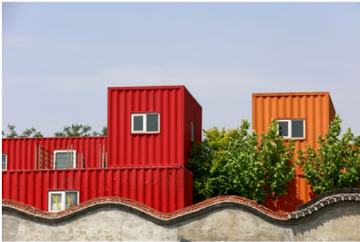
Western Modern Prefab Technology
